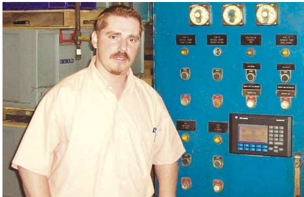
C.R. Hudgins Plant Manager Bobby Robbins stands at the control panel of the company's new zinc plating line.
